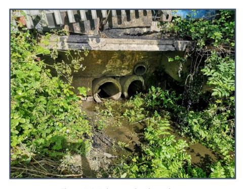
Figure 5-8 Inlet to twin-pipe culvert
